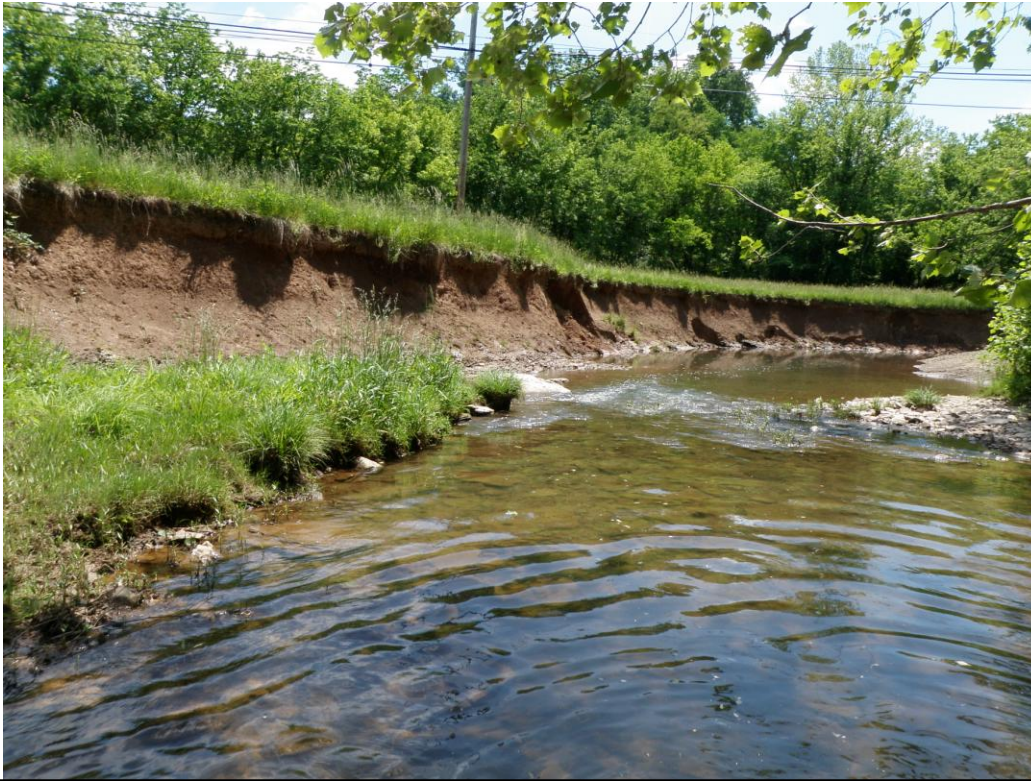
Station OMI-47 – Downstream view of bend on Fatora Property.
