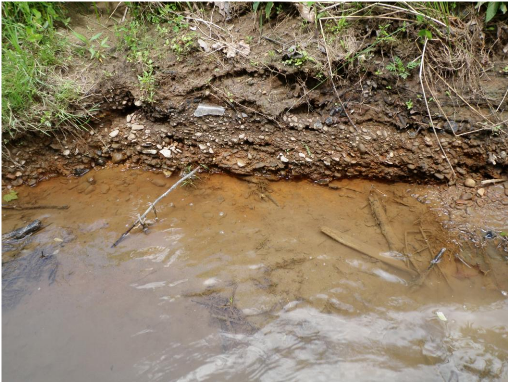
Station OMI-47-(2.7) – Iron precipitates on right descending side.
